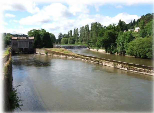
Figure 10 : Barrage de Brieux (Source : Geobs)
